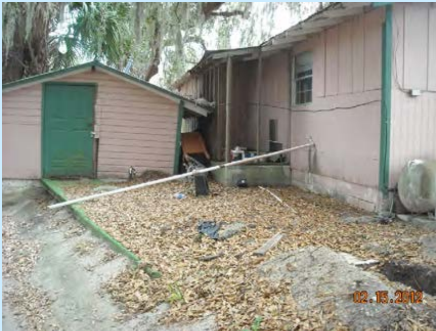
Washing machine discharge
