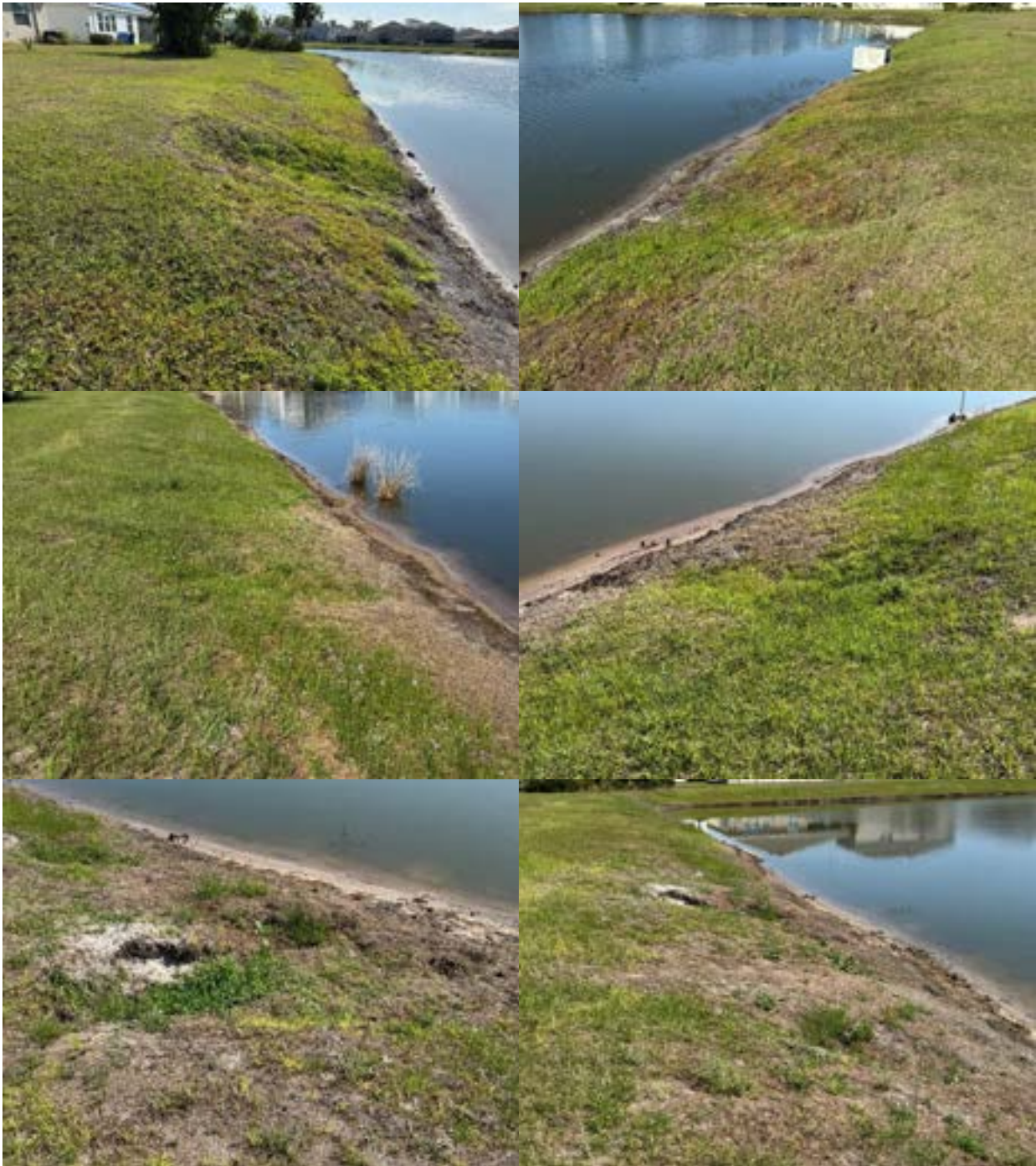
Photo 1- Displays images of the erosion occurring at Pond D.
