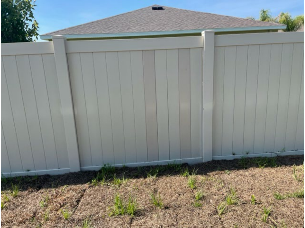
Two fence slats replaced.
