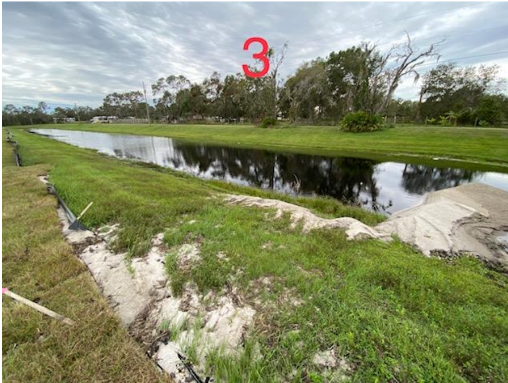
Pond 3 (above) Observed moderate torpedo grass and washout from roadside ditch.
